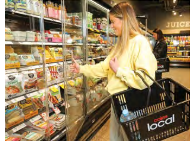
Doors on refrigeration units help to reduce energy consumption.
