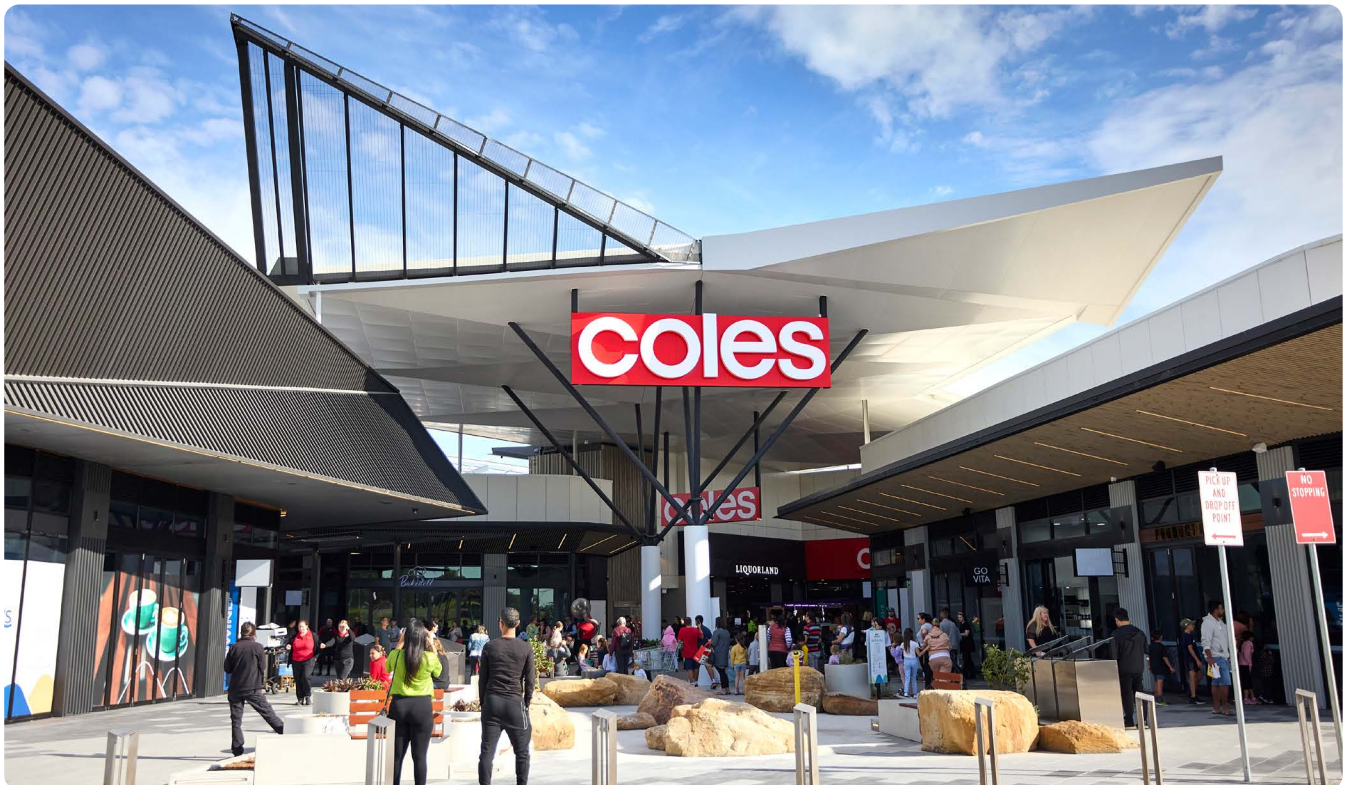
Pictured: Newly opened Coles Box Hill, NSW.
